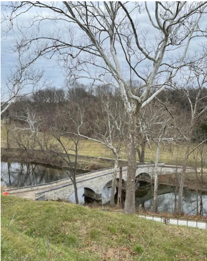
Burnside Bridge, Craig Moore photo
